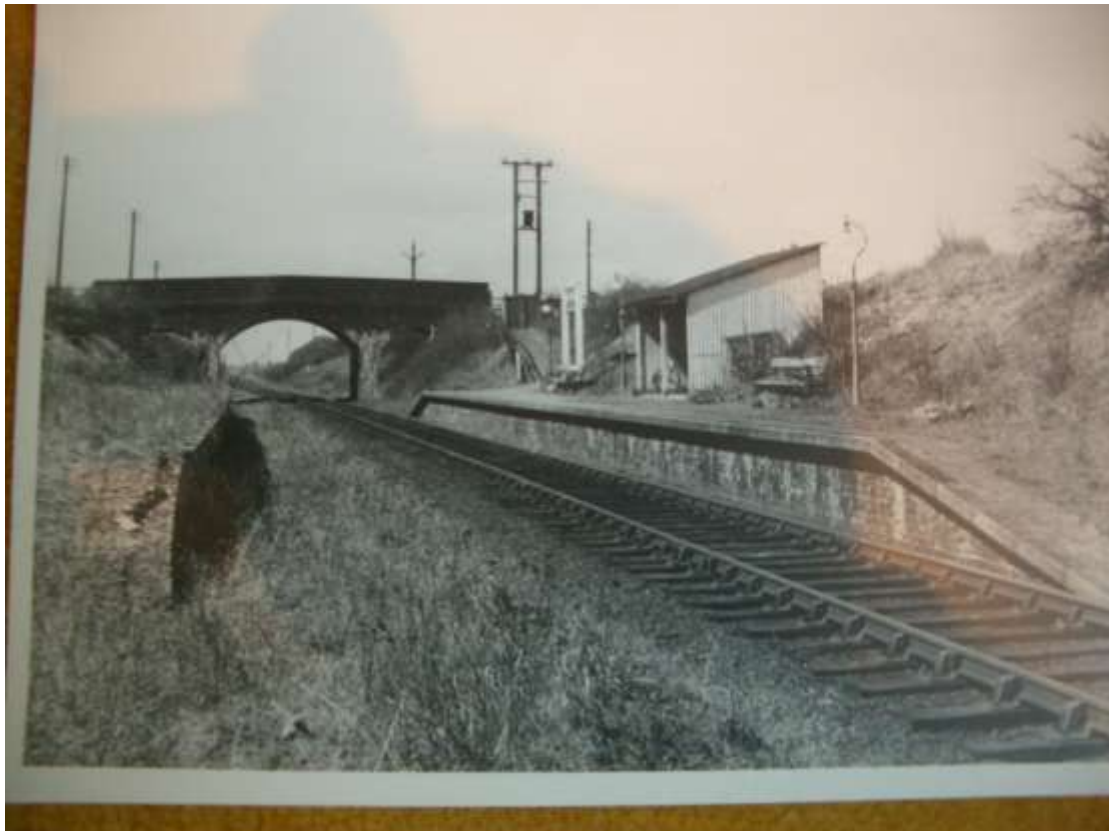
East Halton just before closure. Passing loop removed.
